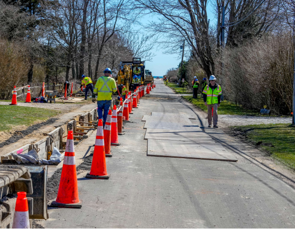
South Fork Wind construction on Beach Lane in East Hampton, NY
